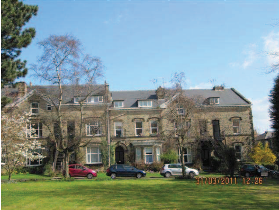
Photo of Previously Existing Bargeboarding and Guttering
